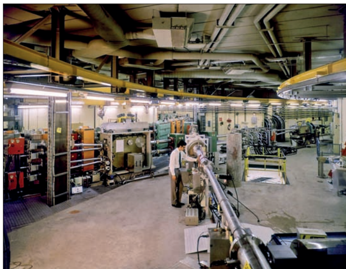
Fig. 2. PSB injection (50 MeV) and transfer (1.4 GeV) lines. The beam coming from the linac (foreground) is distributed vertically to the four PSB levels. After acceleration, the four beams are recombined and transferred (from left to right in the picture) to the PS or ISOLDE.
